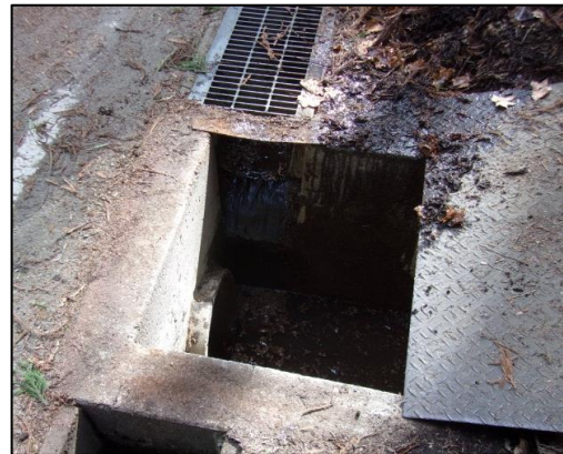
図4:側溝清掃後②
