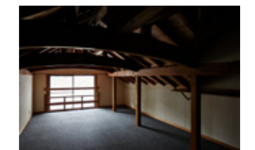
▲ Attic: it uses a traditional Japanese roof framing technique called wagoya.
