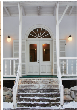
▲ The original entrance is still in use today.
