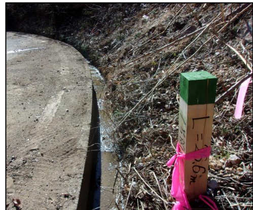
図4:側溝清掃後②
