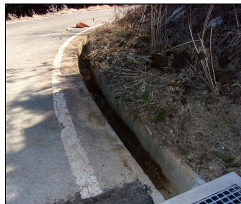
図6:側溝清掃後③
