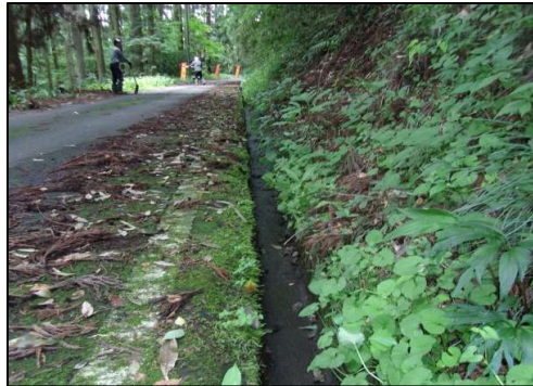
図4:側溝清掃後②
