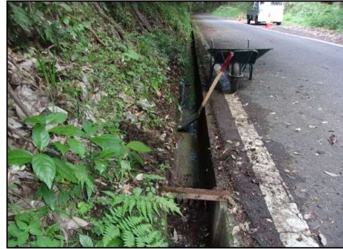
図2:側溝清掃後②
