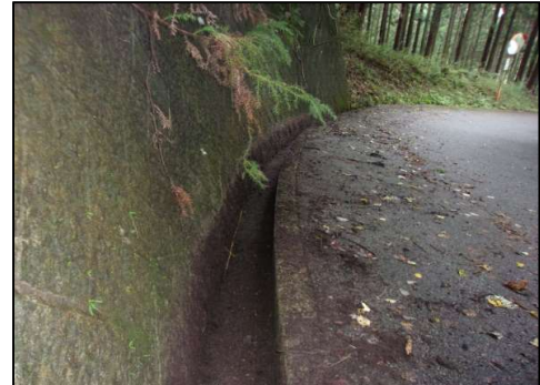
図4: 側溝清掃後②
