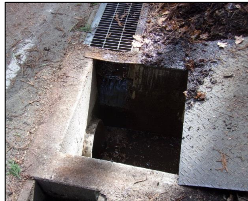
図4:側溝清掃後②
