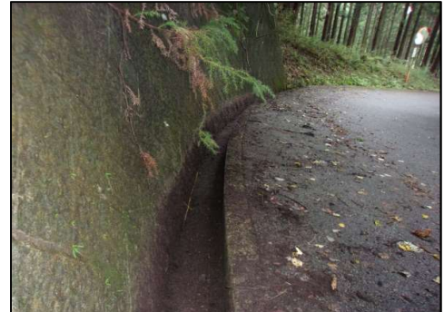
図4:側溝清掃後②
