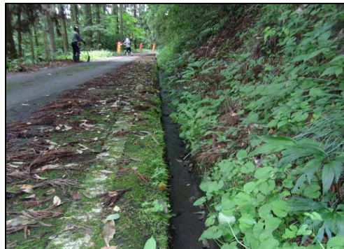
図4: 側溝清掃後②
